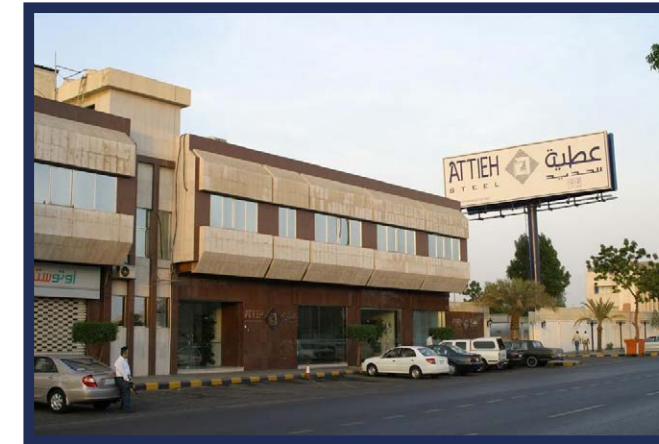
Attieh Trading Company warehouses for Steel industries
