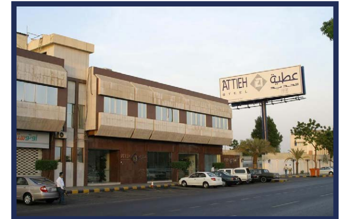
Attieh Trading Company warehouses for Steel industries
