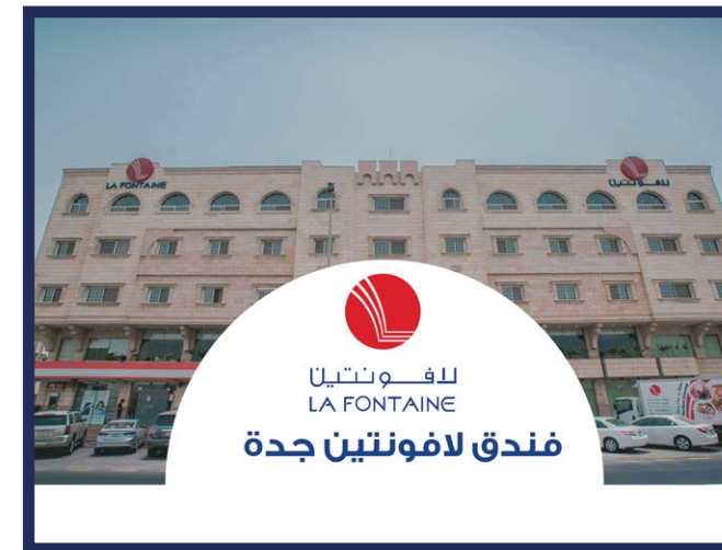
LaFontaine Jeddah Hotel
